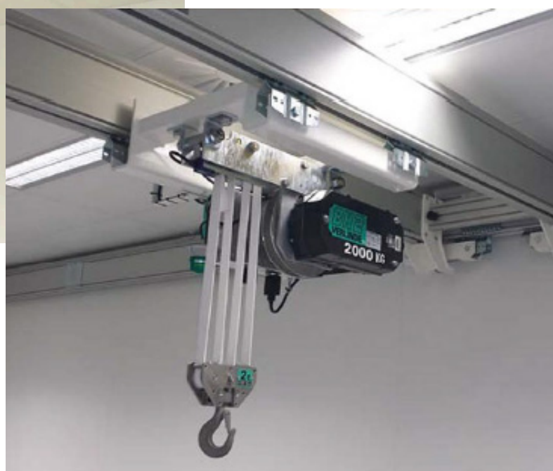
EUROLIFT BH Electric belt hoist on double girder trolley in an EUROSISTEM ALU profile. Option : stainless steel hook block, galvanized body and white belt).
